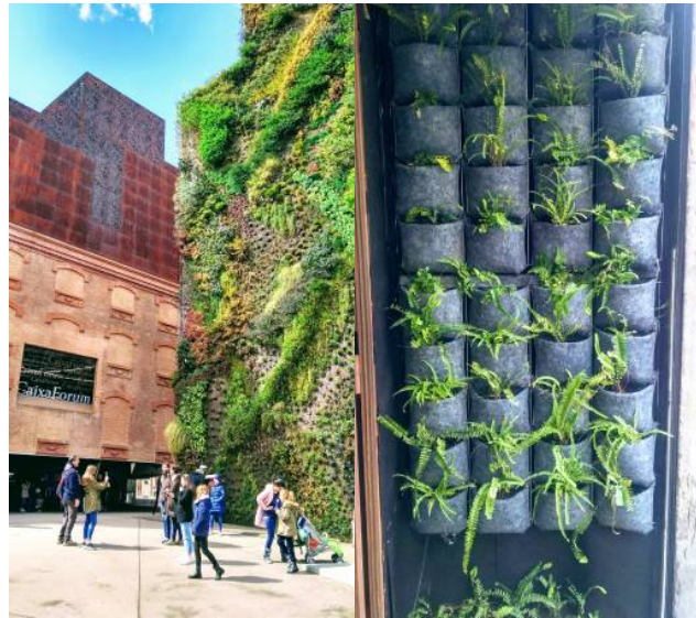
Figure 2: CaixaForum building in Madrid, Spain (Photo by: Szymon Błaszczuk)
